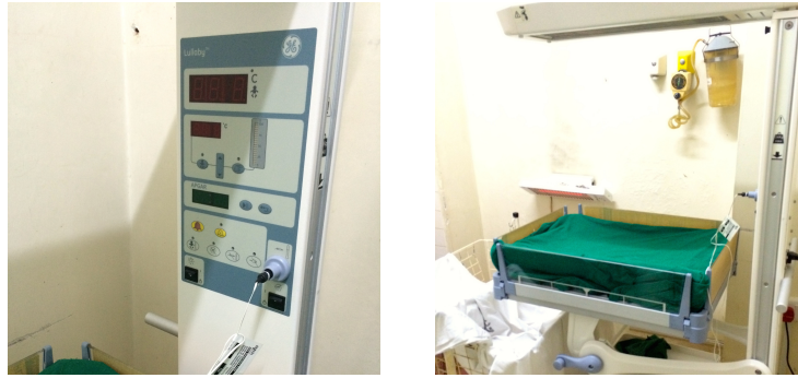
Figure 3.12: Left: Infant Warmer at KCMC Maternity Ward. Right: The skin temperature sensor had been placed below the machine, causing the system to overheat.
