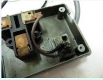
(1) CPAP not working (twice) because plugged into 1 of 3 broken outlets on power strip
