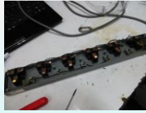
(2) 2 switches show signs of fire; wire outlets directly to avoid switches
