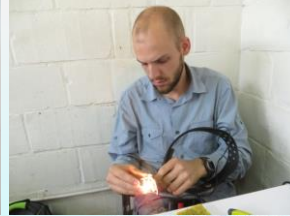
(3) Working again after soldering live wire and strengthening ground bar
