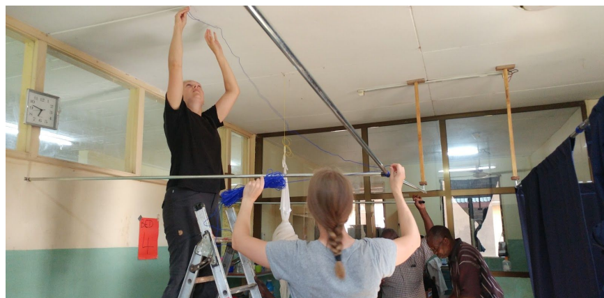
Installing the Pipes for the Curtains
