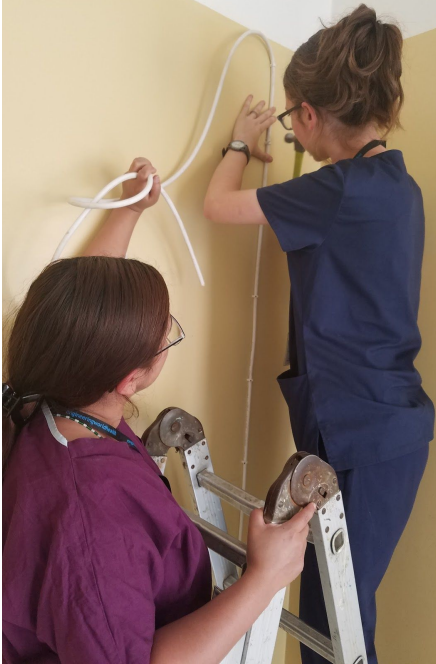
Installing Electrical Line
