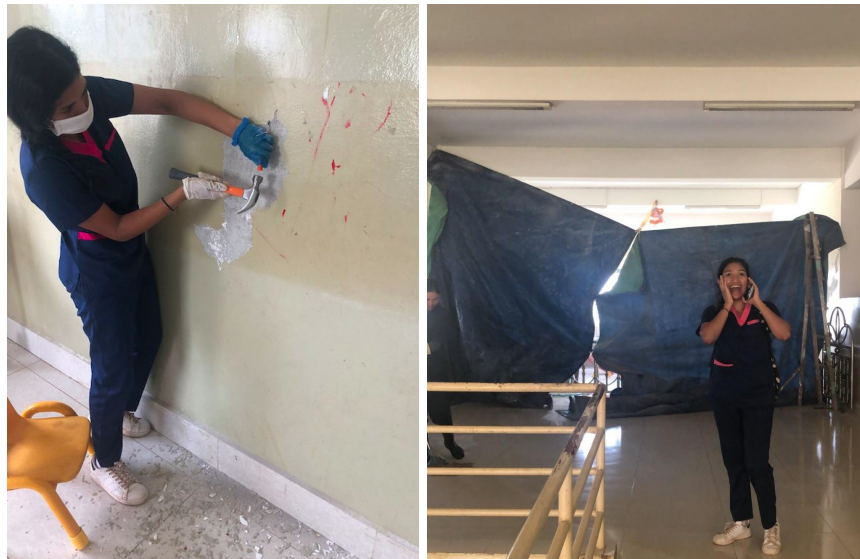
Manually chipping off old and cracked paint; the renovators arrive
