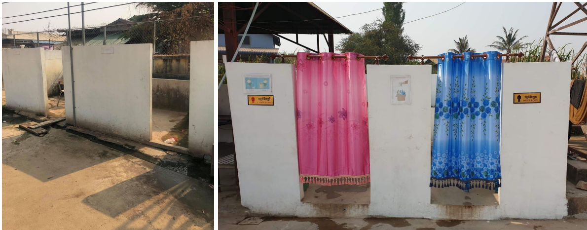
Shower area before; and after
