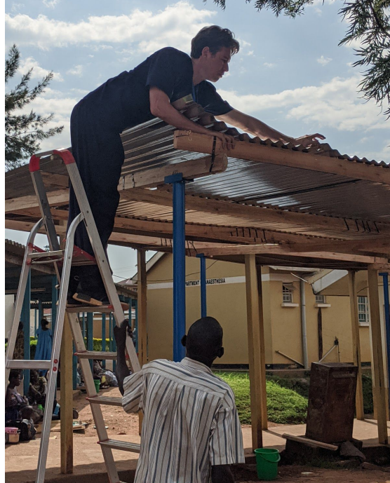
Participant installing the roofing
