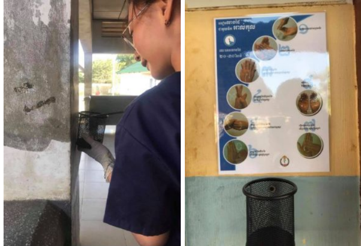
Installing the stations and the finished product
