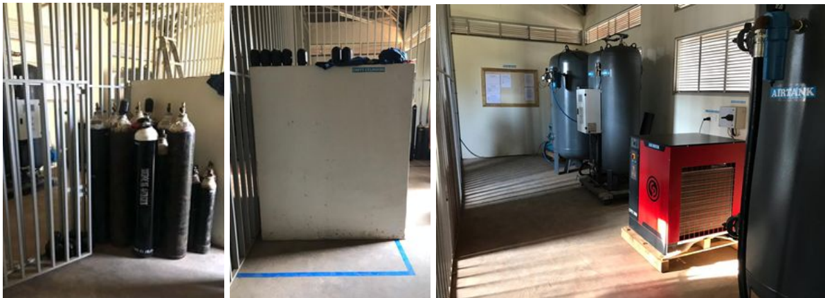
Oxygen plant after secondary project: labels on all tanks and machinery, including on outlets.
