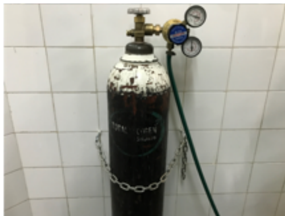
Cylinder secured to wall
