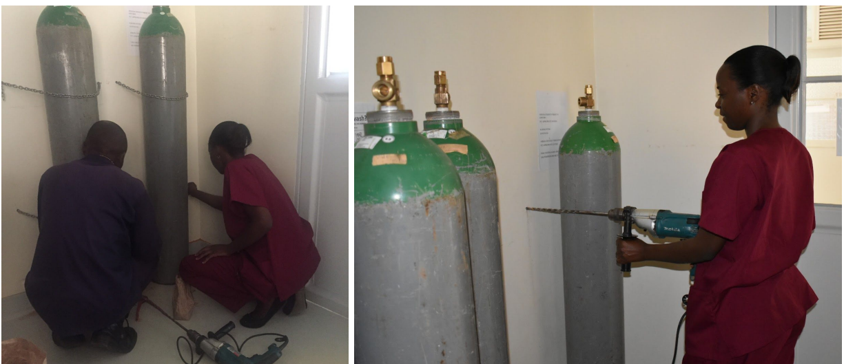
Hospital BMET and EWH Participant securing cylinders; EWH Participant installing chains
