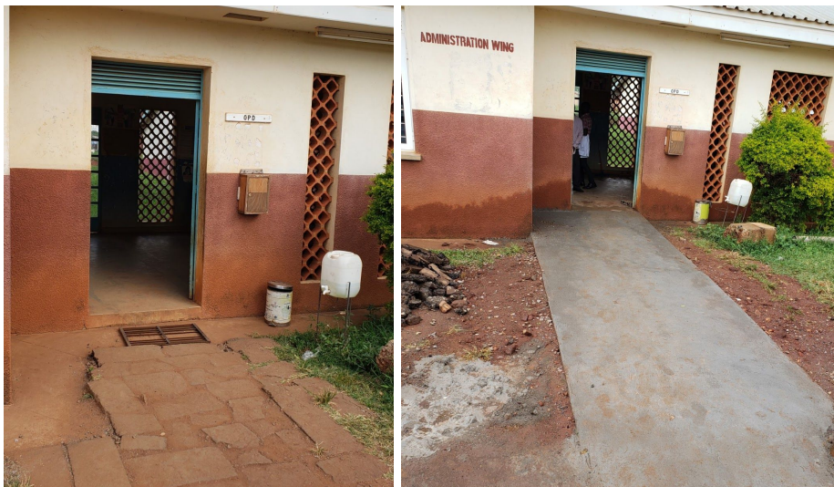
Before and After Ramp Installation
