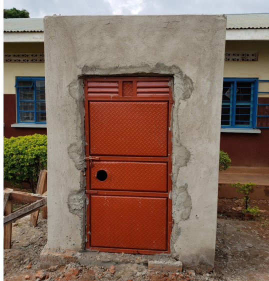
Generator Housing Area
