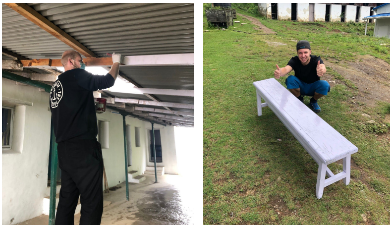
Painting in progress
